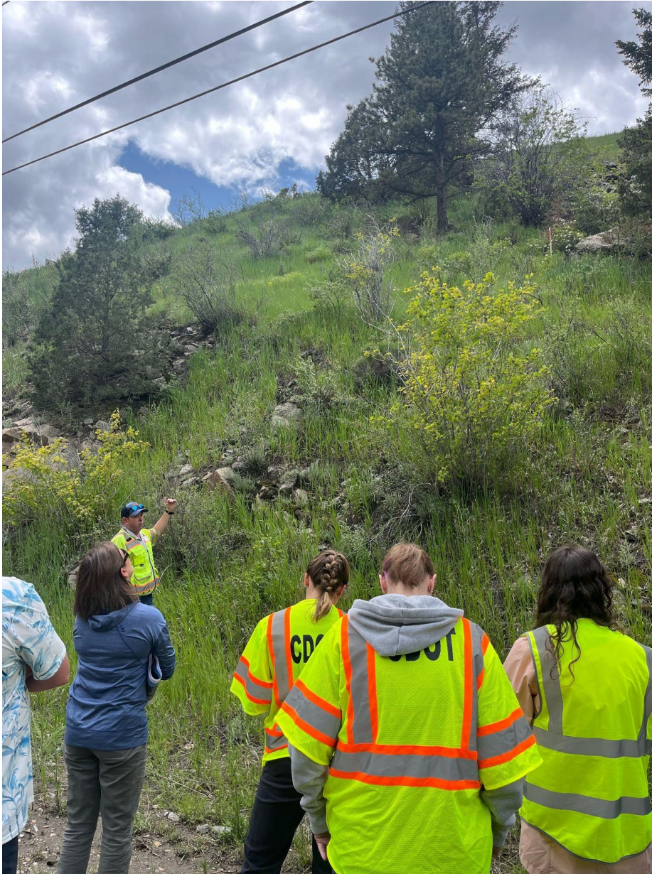
(Pictured Above: Matt Hogan describing location of New Access Road and adjacent Retaining Wall to access pier locations for Bridge A- example indicated by pink stake up the hill)
